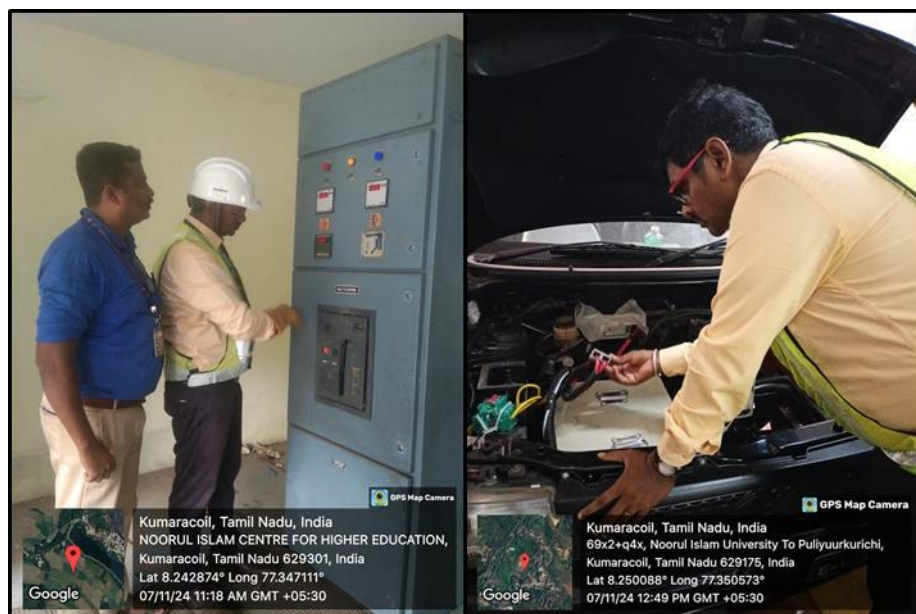
Energy conservation facilities observed in the Campus
